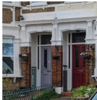
Right: Doorway detail, showing the glazed tiles
